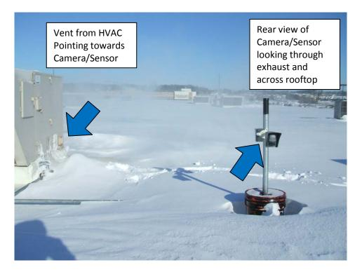
Moreover, the camera that had not been active was pointed at the adjacent rooftop. It had been installed such that the motion sensor should not trip because of activity on the adjacent roof.
